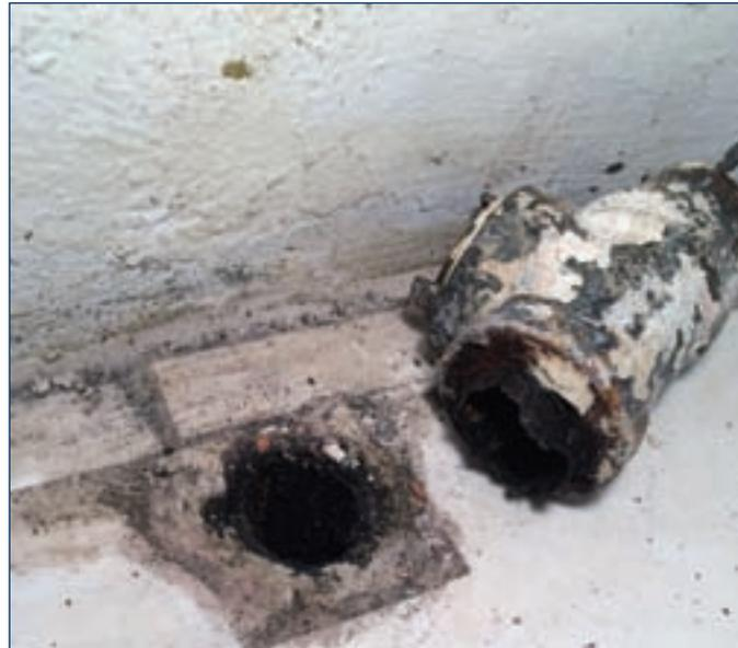
Corroded wet return snapped off at floor.
