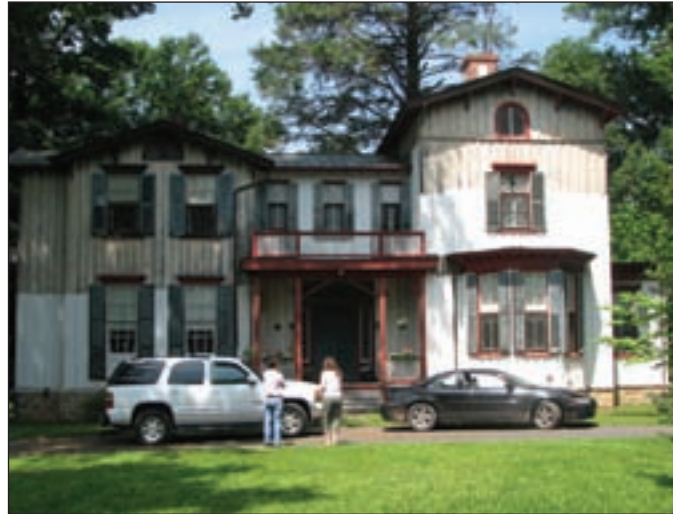
Photo 4: The second project was in an Italianate farmhouse built in 1860. The house is located in Thurmont, Md., about an hour north of the city, and is still in the same family as the original owner.
