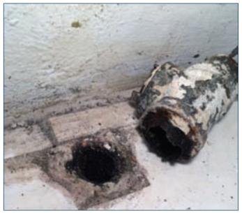
Corroded wet return snapped off at floor.
