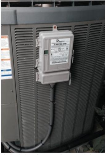
The client had elected to have a utility company load shedding device, as pictured here. In exchange for a lower electric bill, the utility can shut off the AC unit during peak electrical demand.
