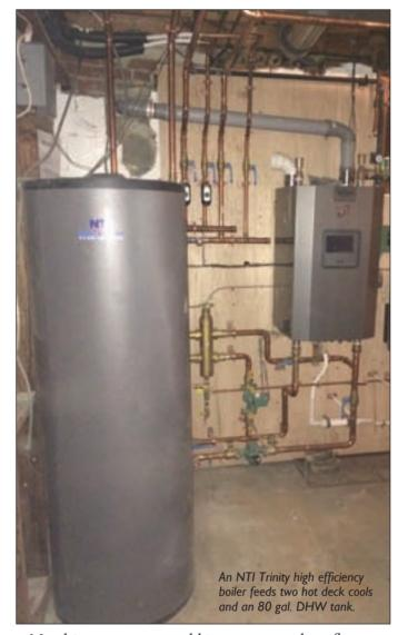
My ultimate system would incorporate radiant floor heat, panel radiators and wall-mounted towel warmers. Unfortunately, the budget did not allow for this. We settled for the next best thing: a hydronic system powered by an NTI Trinity 95 percent AFUE modulating condensing gas, wall-mounted gas-fired boiler (See photo). We dropped a PPS flexible liner down the old boiler flue and vented it through the roof.
