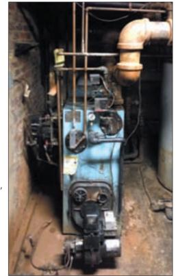
*Photo 2:* The system was burning almost \$3,000 worth of oil per month, and was performing poorly with water hammer, unbalanced heat, short cycling lock-outs and poor reliability.
