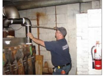
Lead technician Brian Golden fabricating one of the header risers in the V-9 steam boiler.
