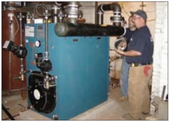
*Brian Golden finishing up the drop header on the Burnham V-9 steam boiler.*
