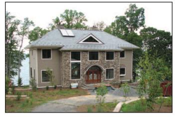
Horbaly Residence located in Montross, Va. overlooks the Potomac River. Two Viessmann Vitosol flat panel solar collectors are mounted on the upper left portion of the roof.
