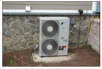
An Altherma outdoor unit is mounted on concrete base pad.
