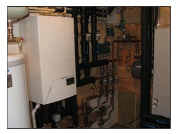
An Altherma Hydrobox mounted on mechanical room wall.
