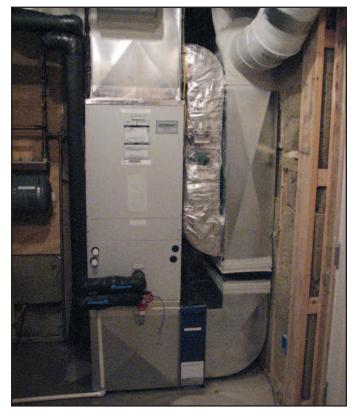
The Altherma system supplies hot and chilled water to this variable speed air handler.
