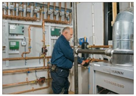
Mechanic Papa Duric completes a connection for the system's Caleffi hydro-separator.
