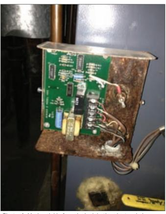
Photo 4: Mark quickly found a leak in the electronic low water cutoff probe that shorted out the circuit board.
