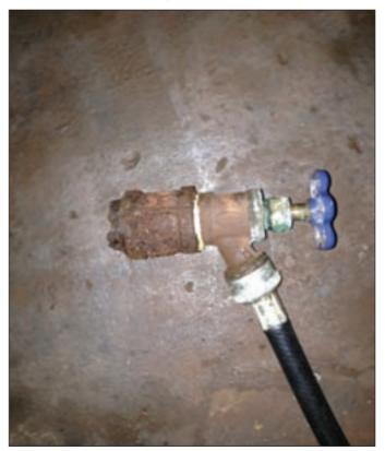
Photo 2: The boiler drain was extended beyond the boiler jacket by a 3/4-inch black nipple and coupling. It had been leaking for some time and caused the nipple to corrode.
