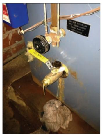
Photo 3: Mark removed the stub with an easy-out and a 24-inch wrench. He then chased the threads with a pipe tap and threaded a new brass nipple and ball valve with a hose end.
