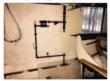
Boiler feed pumps can do a great job of maintaining a steady water line, especially if the new boiler does not hold as much water as the older boiler it replaced. It can store condensate and pump it into the boiler as needed, preventing the burner from shutting off on low water.
