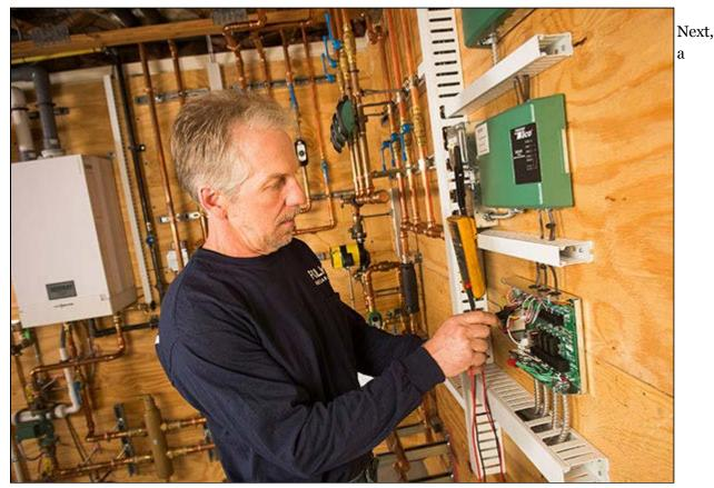
Viessmann Vitodens condensing gas boiler was piped in, sending priority heat to an 80-gal. stainless steel indirect water heater, which provides for all of the domestic hot water needs.
