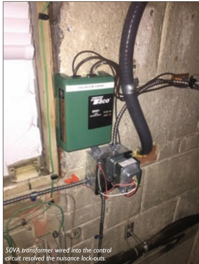
50VA transformer wired into the control circuit resolved the nuisance lock-outs.
