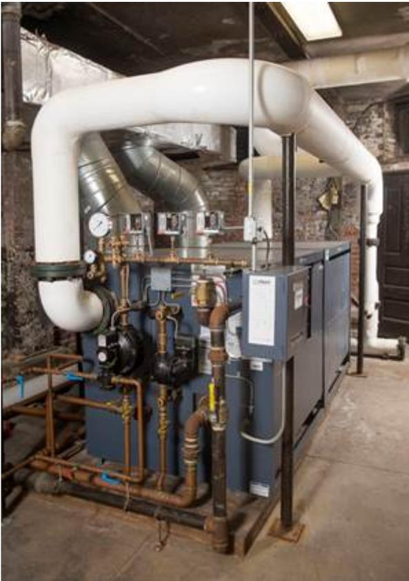
*Installing a Weil-McLain LGB-20 atmospheric draft steam boiler improved resident comfort and offered major energy savings for the Mendota. Boiler Replacement Full Steam Ahead*
