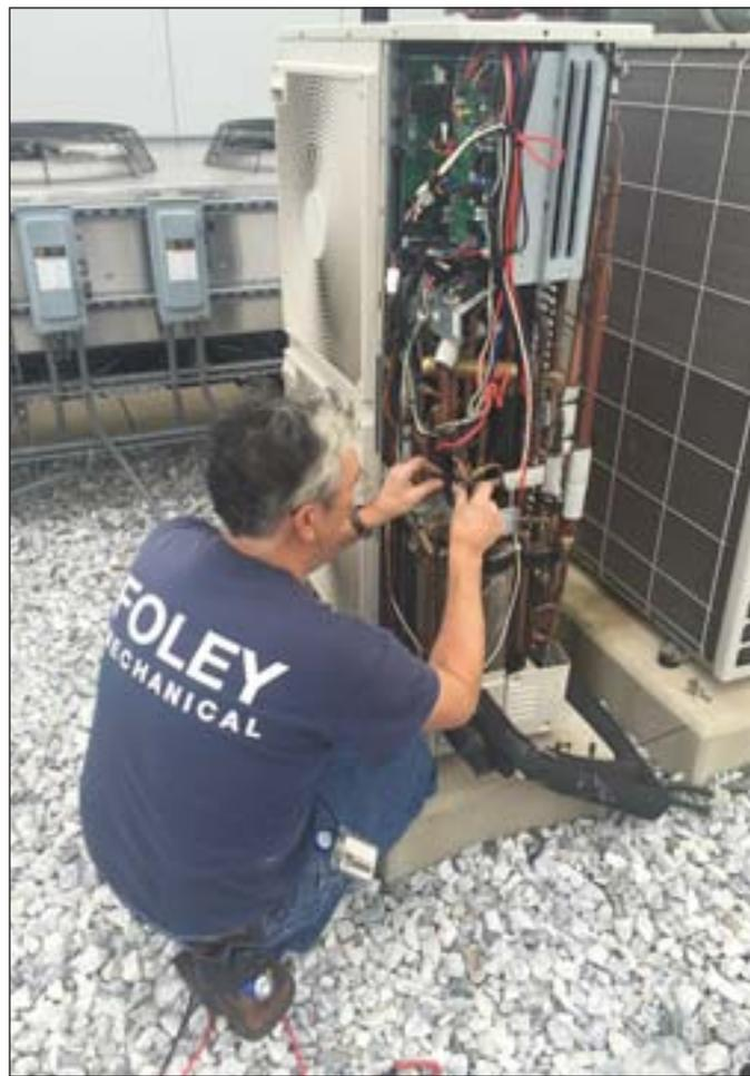
Foley Mechanical Service Technician Mark Wilson replacing the discharge temperature sensor.
