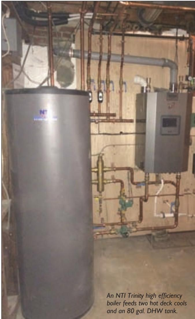
An NTI Trinity high efficiency boiler feeds two hot deck coils and an 80 gal. DHW tank.
