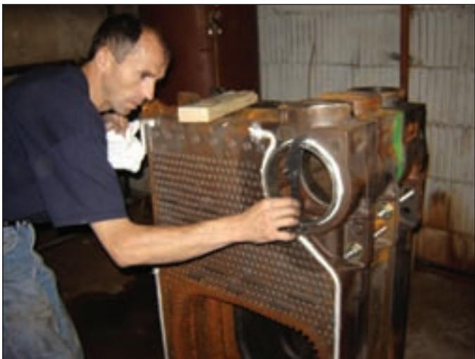
*Foley Mechanical technician using a gauge to check the steel push nipples in the cast iron boiler sections.*
