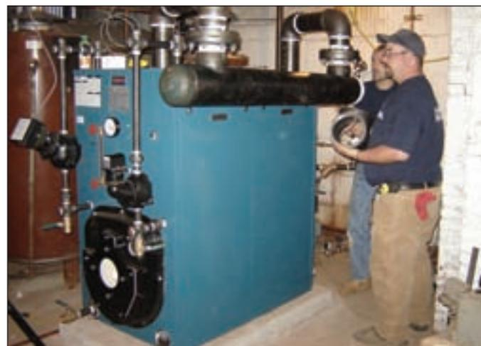
Brian Golden finishing up the drop header on the Burnham V-9 steam boiler.
