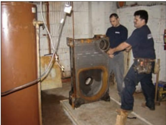
*Foley Mechanical technicians assembling V-9 cast iron steam boiler sections.*
