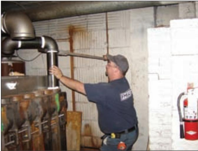
Lead technician Brian Golden fabricating one of the header risers in the V-9 steam boiler.
