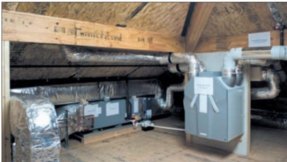
*For passive homes that "you could heat with a candle," adequate ventilation is paramount. In this installation two ERVs run continuously, but the air system incorporates an experimental ground loop to temper the incoming fresh air.*
