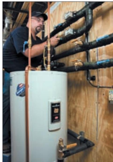
*Foley technician, Brian Golden, adjusts a system that incorporates two 50-gallon Bradford White water heaters behind the preheat tank.*
