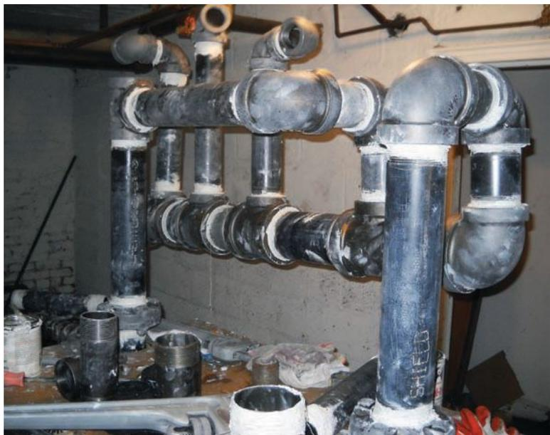
Because of his location in New York, Shay is called to work on many old steam and hot water systems. Shown here is a small boiler steam header.
