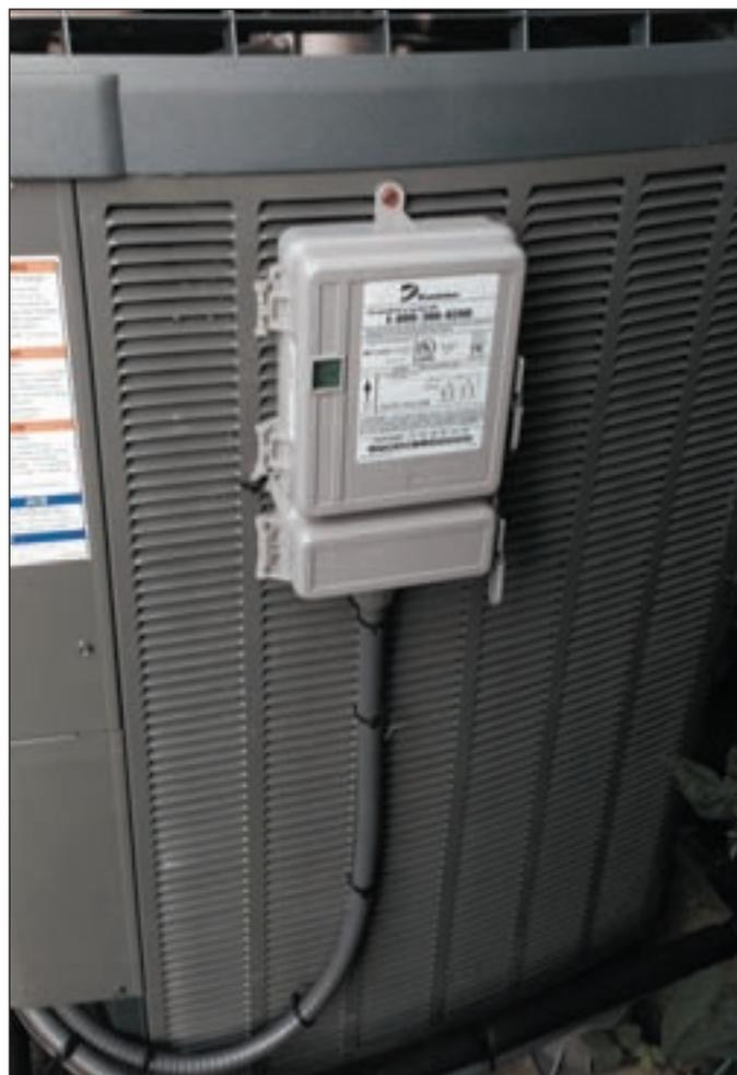
*The client had elected to have a utility company load shedding device, as pictured here. In exchange for a lower electric bill, the utility can shut off the AC unit during peak electrical demand.*
