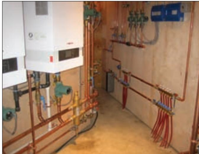
Boiler replacement project in Frederick, Md., featuring a Sorbox hydronic filter tied to existing basement slab radiant system.
