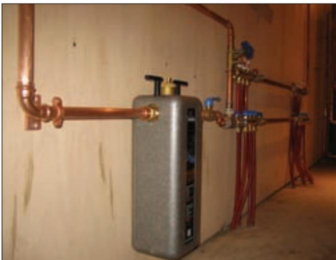
Sorbox filter installed in hydronic radiant system with bypass, balance and isolation valves.
