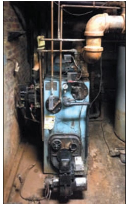
*Photo 2: The system was burning almost \$3,000 worth of oil per month, and was performing poorly with water hammer, unbalanced heat, short cycling lock-outs and poor reliability.*
