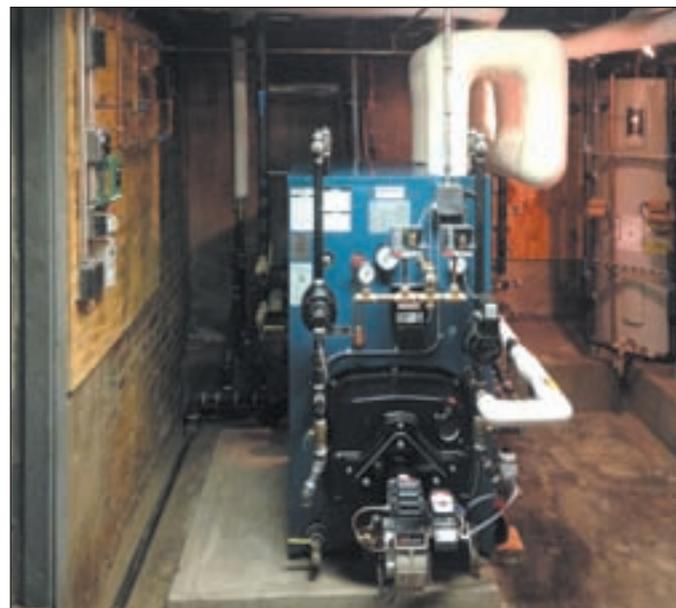
*Much better! A Burnham V-904 boiler was sized to the connected radiator load and fired with a Beckett CF800 burner. A motorized combustion air damper that closed during the off cycle eliminated an open window.*
