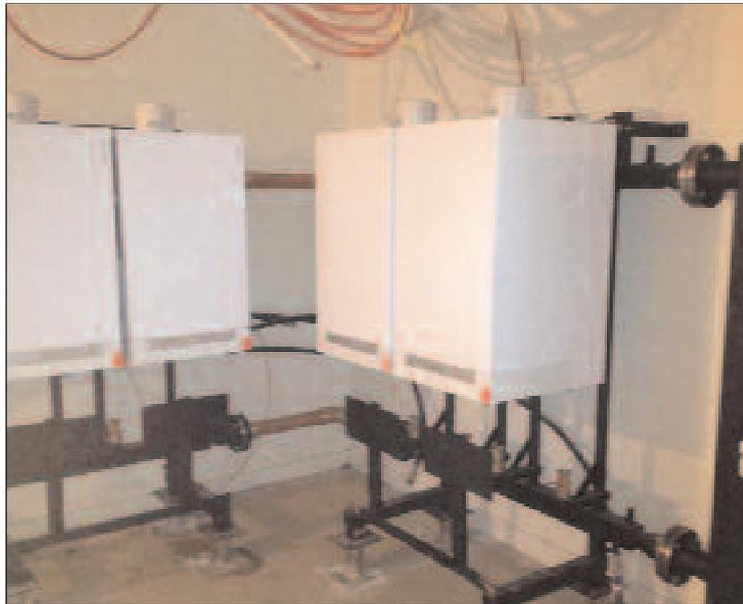
*The Viessmann rack packs a little over 1.5M BTU/hr. into the corner of a very tight mechanical room.*
