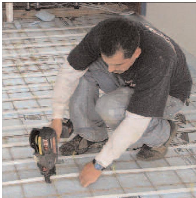
Foley Mechanical technician Joe Guerrero uses the MAX tie tool to attach radiant tubing to steel mesh.
