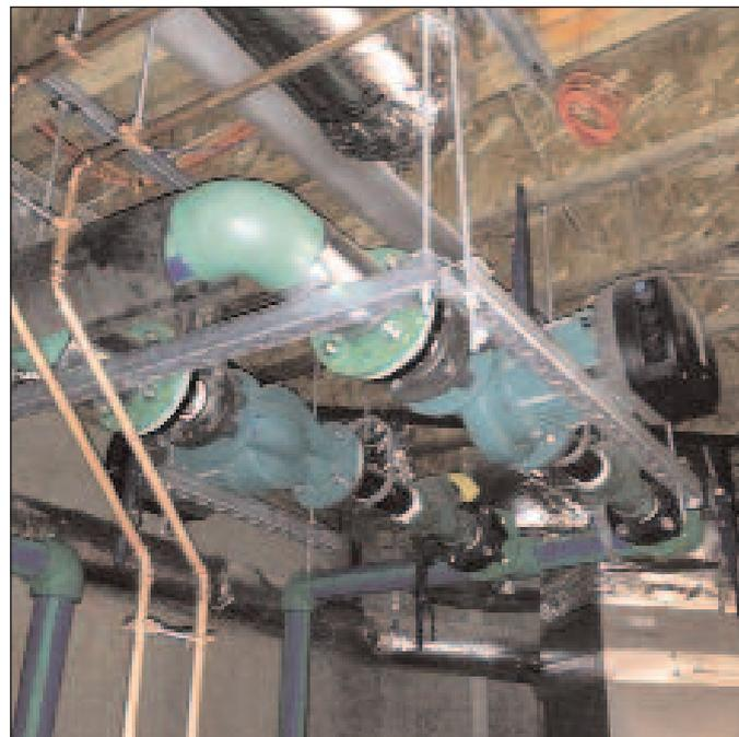
*The Aquatherm fusion welded polypropylene system installed in a geo loop application delivers reliability at a cost significantly less than L copper.*
