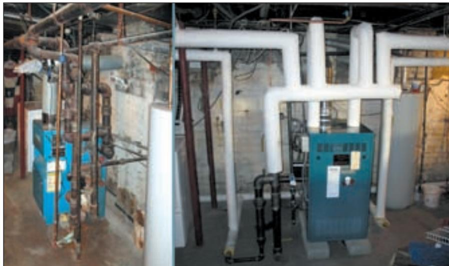
Before (left) and after: A messy, old, patched-up and screwed-up Hutchinson 2-pipe steam system gets a new lease on life with proper rebuilding and a few upgrades to restore it so it would operate to its original excellent levels.
