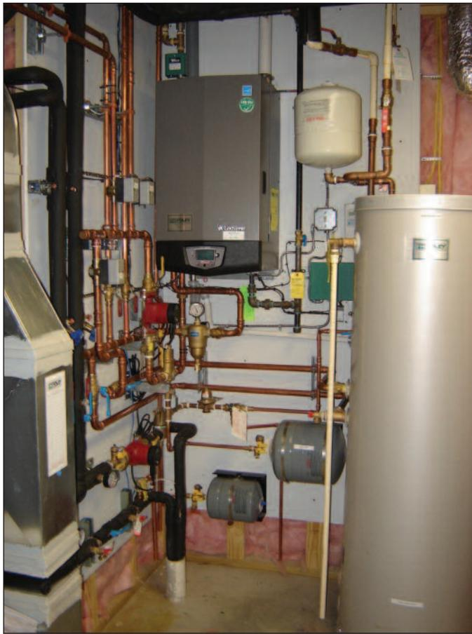
The heat source is a Lochinvar Knight WHN055 wall-mounted condensing gas boiler (96% AFUE). This boiler has a low pressure drop fire tube heat exchanger and can modulate from 11–55 K Btu input. The low pressure drop also allowed the system to operate with only one Grundfos Alpha pump that only draws approximately 18 watts at design conditions.
