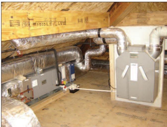
All duct runs were sealed with mastic and insulated with R-8 foil-faced duct wrap, and were as short as possible.
