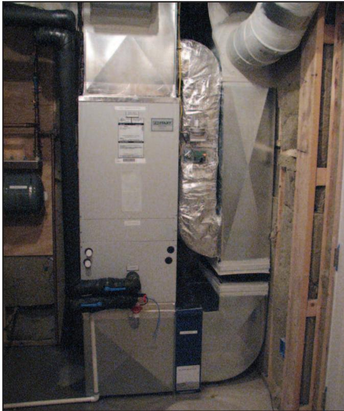
The Altherma system supplies hot and chilled water to this variable speed air handler.
