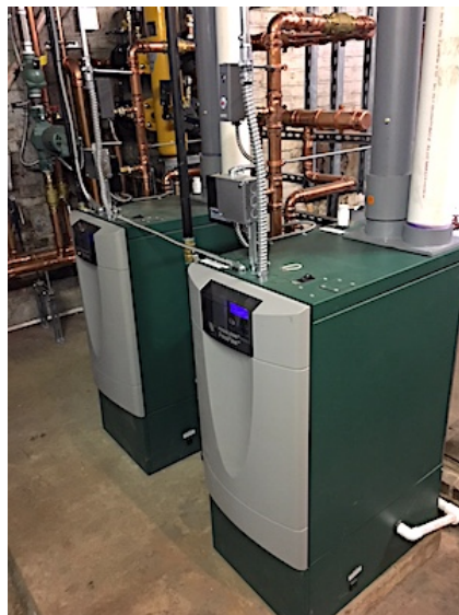
Recently completed project; before piping was insulated.
