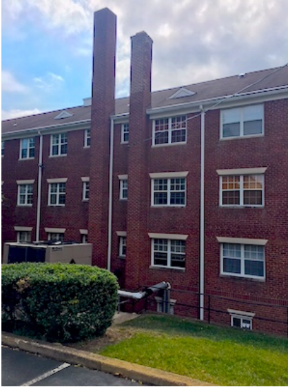
The 1950s apartment building in Arlington, Va. gets a mechanical upgrade.
