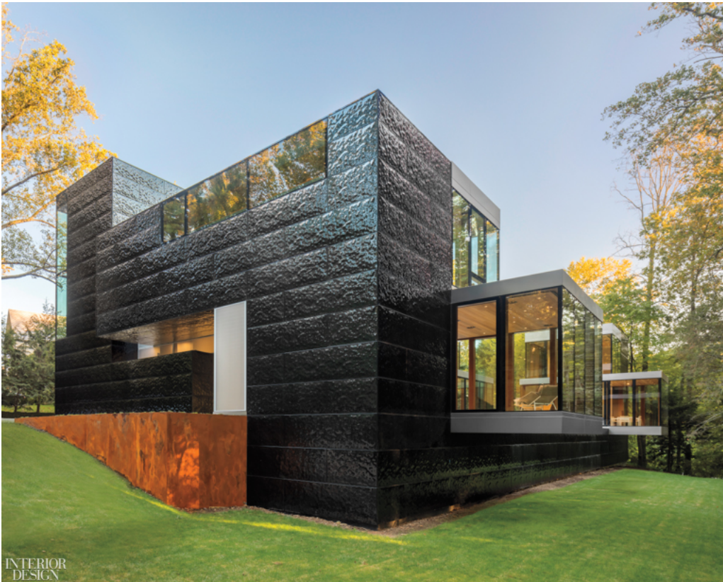
Crisp glazed volumes pop from the house's rough-hewn stainless-steel facade. Photography by Paul Warchol.
